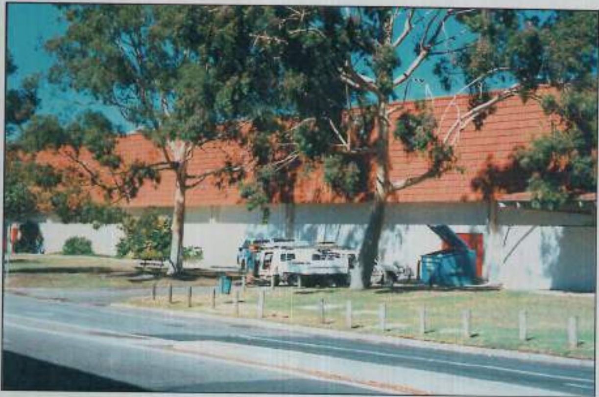
This blank wall up against Helena Street damages pedestrian amenity.
