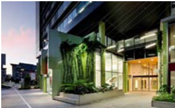
Secondary frontages: clear entries, apertures and articulation are encouraged at ground level
