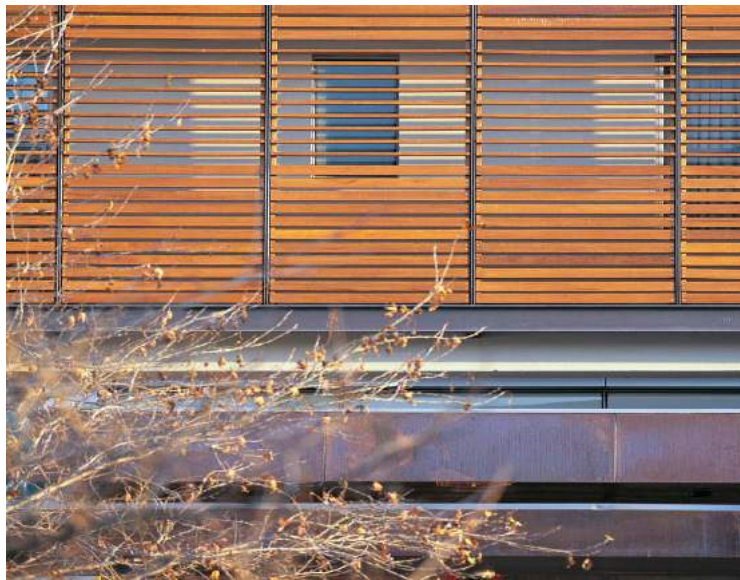
Figure32_Shading devices and double glazing allow for more energy efficient buildings
