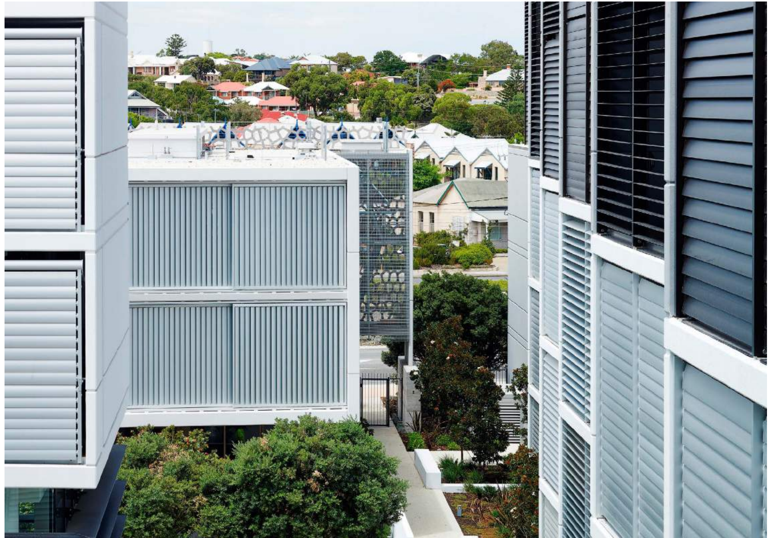
Figure29_Screening elements can be incorporated into a building's architecture to conceal services
