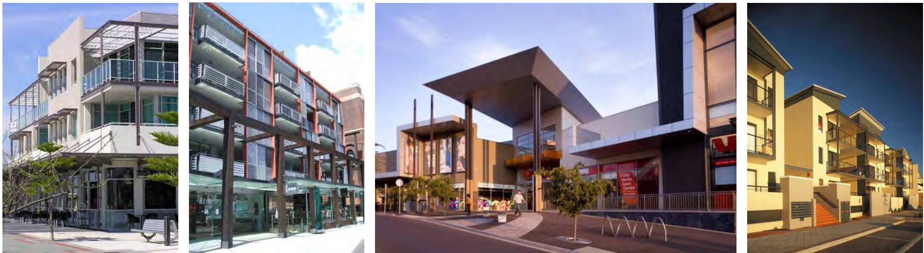
Figure 14_Building setbacks will be consistent with a precinct's intended character; buildings on active streets will be constructed at the property line to promote engagement and commercial interaction with the public realm
