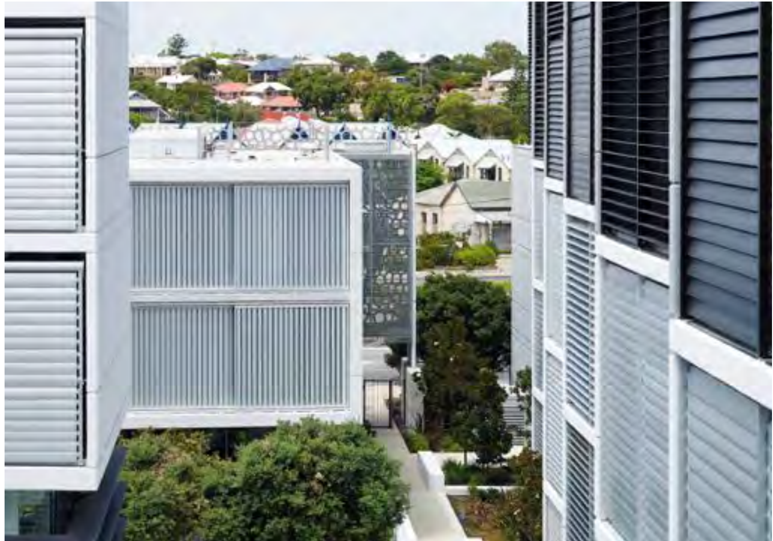
Figure 21_Screening elements can be incorporated into a building's architecture to conceal services
